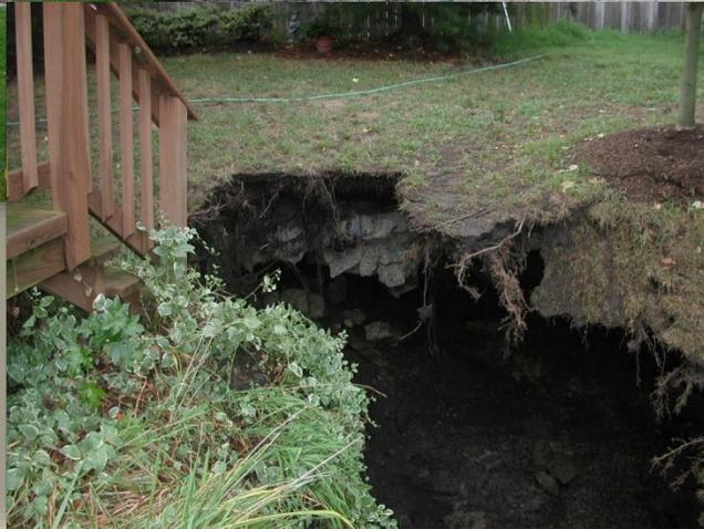
A vertical opening was discovered by DMLR during the inventory process. The property owners were contacted and informed of the AML feature on their property and agreed to have it reclaimed. The vertical opening was filled and capped, and typical marker posts were installed to indicate its location.
