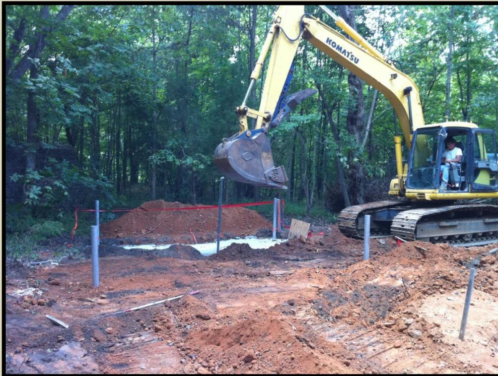
*The contractor is re-grading the reclaimed shaft to the approximate original contour of the land before mining. The area will then be seeded for re-vegetation. Metal posts demarcate the location of the reclaimed shaft.*
