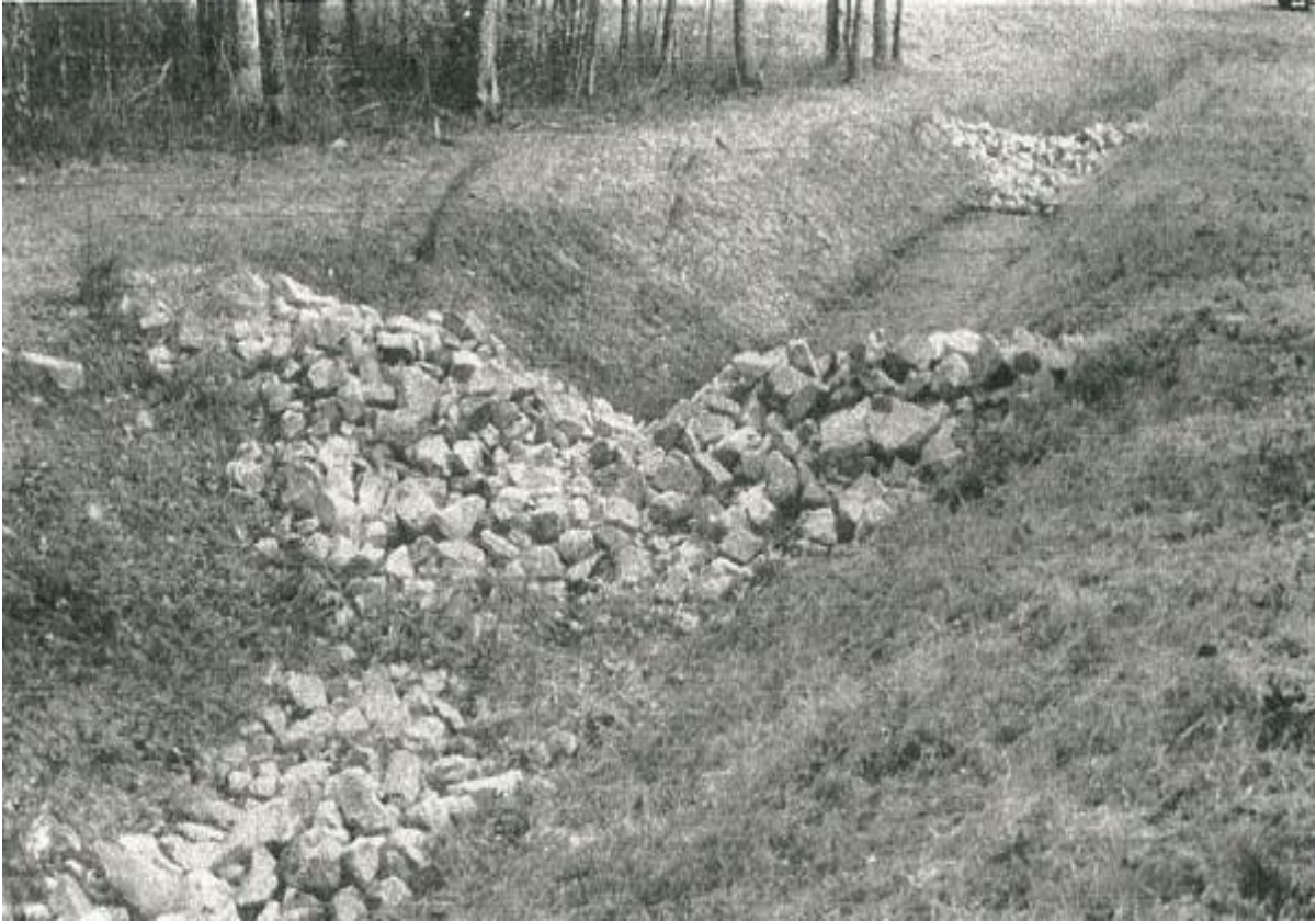
FIGURE 2. Example of a rock check dam
