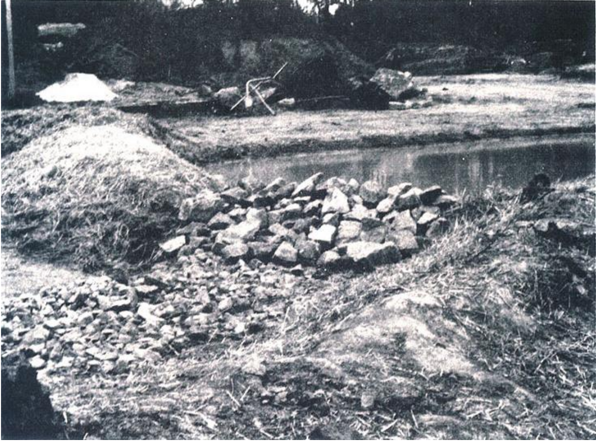
FIGURE 7. Example of temporary sediment trap
