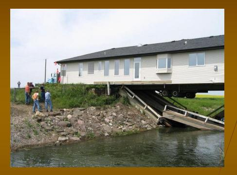
A number of fatalities in recent years have been due to lifting loads that were beyond the capacity of the equipment used. Know the capacities of the equipment you are using and the weight of the load you need to move, lift, etc.
