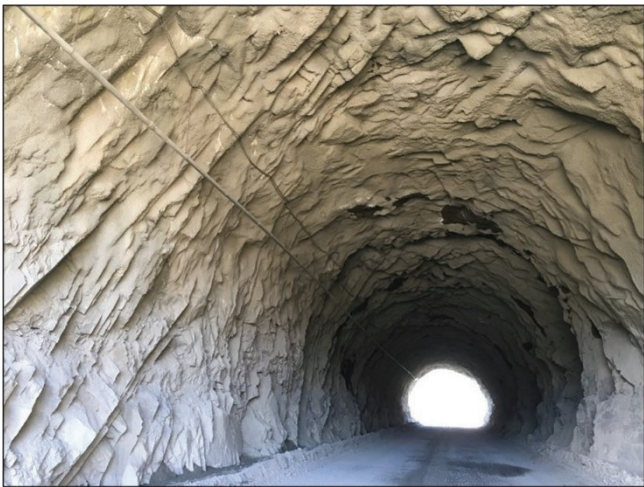
Figure 5 (left): Photo of the completed tunnel connecting the North and South Quarries. Figure 6 (Right): The completed tunnel was large enough to allow haul trucks to pass through to carry stone to the processing plant.
