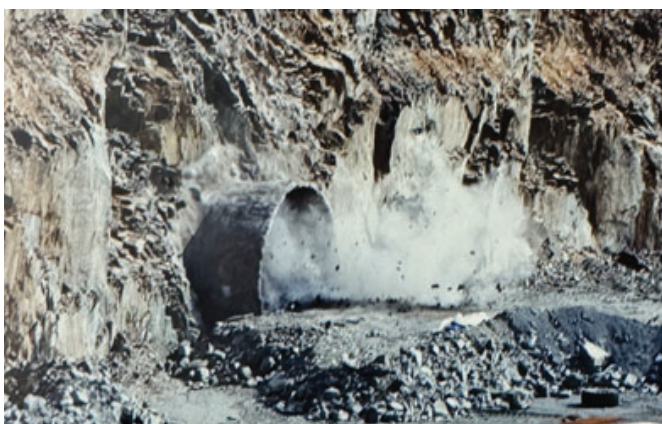
Figure 3 and Figure 4: Photos taken in February 1995 during the tunnel construction. Figure 3 (left) shows a shot taking place to square the face. Figure 4 (right) shows material being mucked from the tunnel during a snowstorm.
