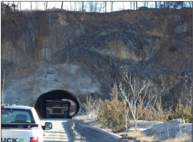
Figure 5 (left): Photo of the completed tunnel connecting the North and South Quarries. Figure 6 (Right): The completed tunnel was large enough to allow haul trucks to pass through to carry stone to the processing plant.
