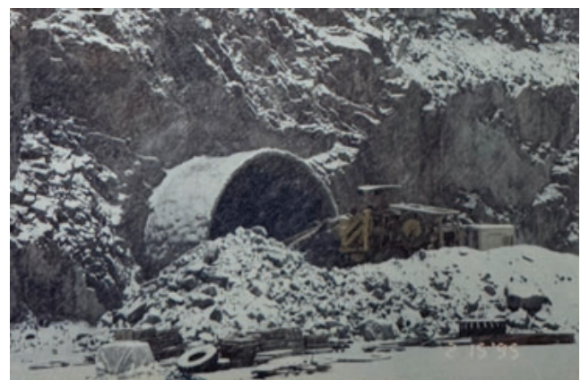
Figure 3 and Figure 4: Photos taken in February 1995 during the tunnel construction. Figure 3 (left) shows a shot taking place to square the face. Figure 4 (right) shows material being mucked from the tunnel during a snowstorm.
