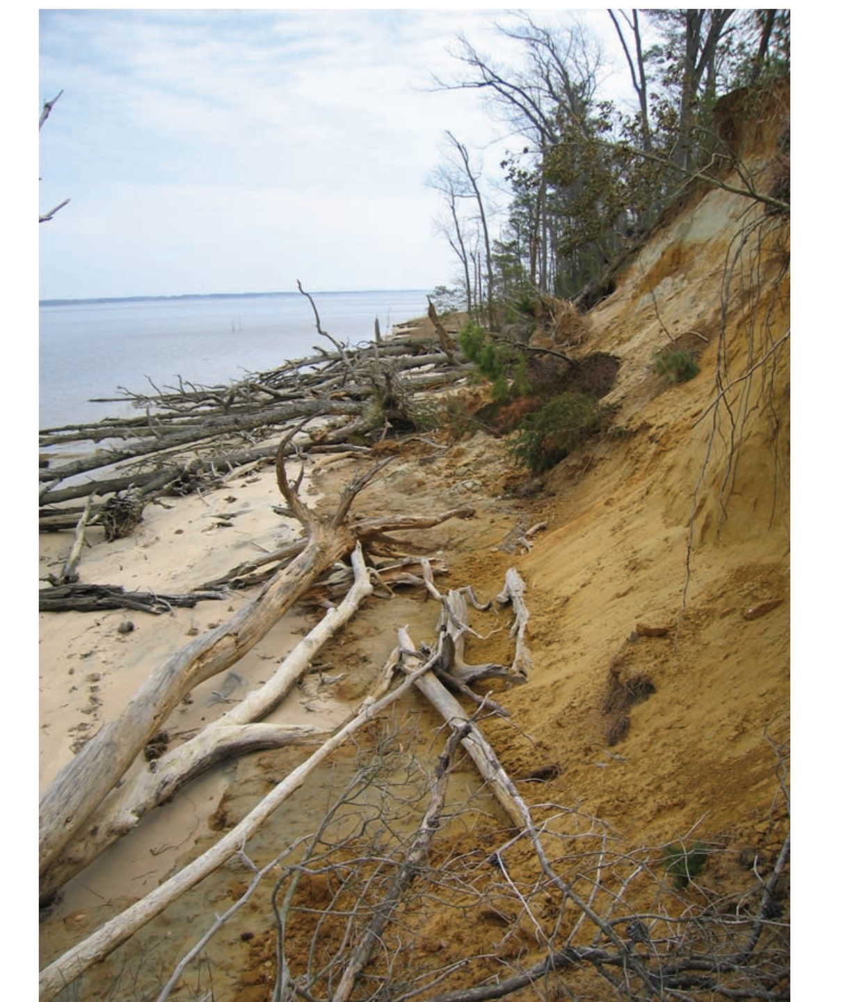
Figure 3. Continuous shoreline erosion at York River State Park.
