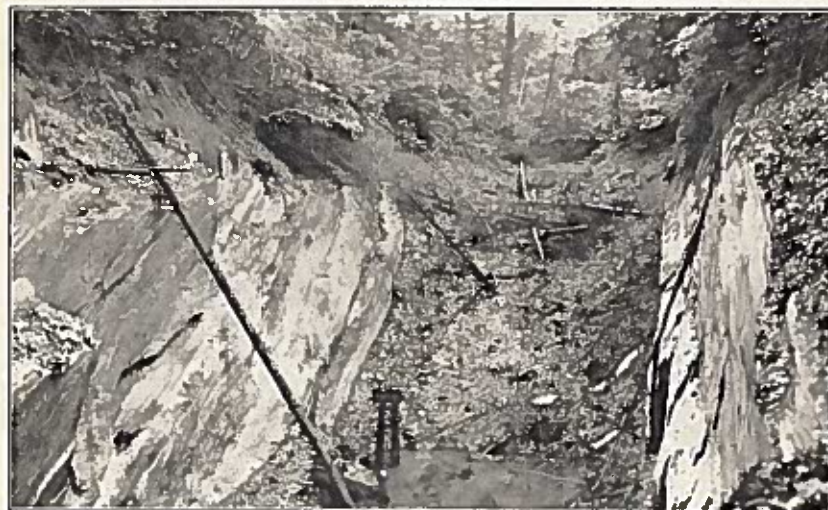
B. Open cut at the Vacluse mine, near south end of area shown on Plate 1.
