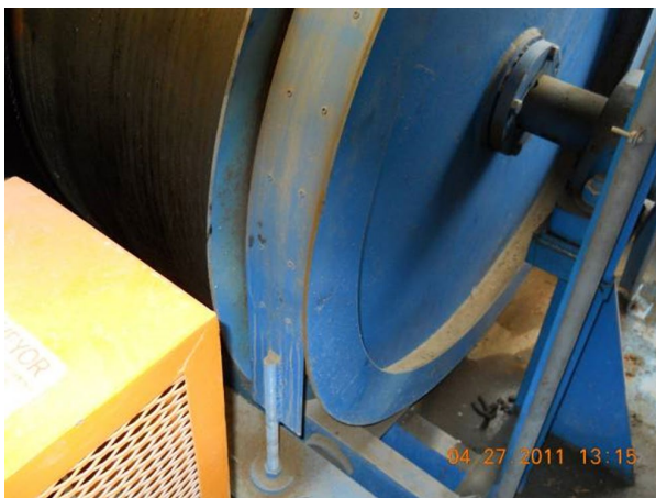
Hydraulic operated brake
