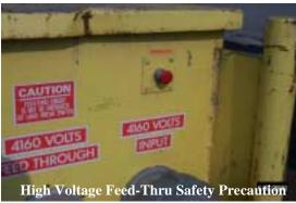
A certified repairman received serious injuries when he contacted one phase of an energized 13,800-volt circuit after failing to de-energize the correct circuit (top left above). Numerous electrical fatalities, serious accidents and near-miss incidents have occurred recently in Virginia and across the nation at coal mines when repairmen failed to identify, de-energize, lock out and ground the correct circuit being repaired.
